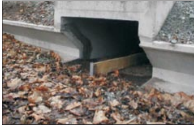
Fig. 6. Tunnels and ZIEGER type guiding fences for amphibians. Maintaining the natural soil and placing a guiding board in the tunnel is significant.
