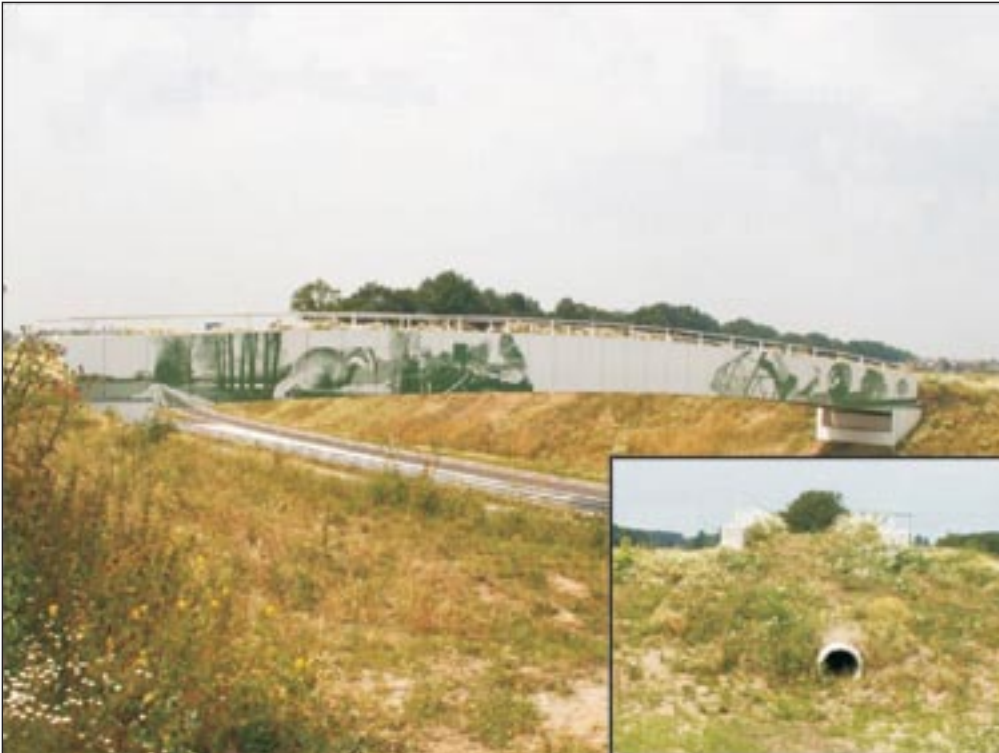
Fig. 6. The ecombiduct is a combination of a (in this case small) ecoduct and a badger tunnel
